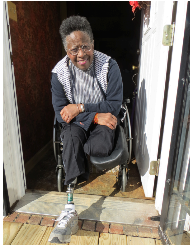
Rosaland watches as Habitat Susquehanna's Repair Program builds an accessibility ramp for her home.
